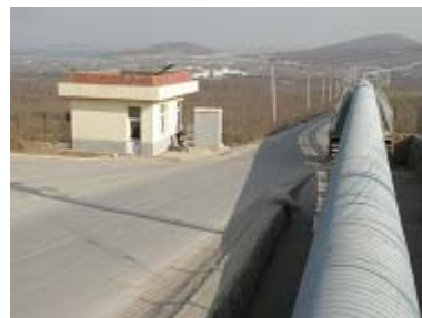
Conveyor for limestone
