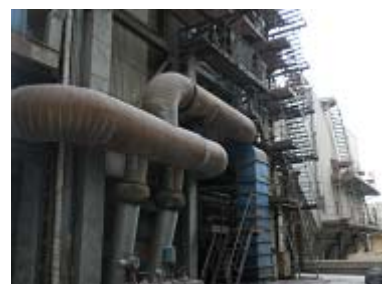
Exterior view of generation facility
