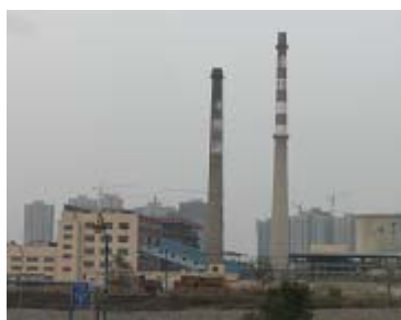
Full view of Yendao Thermal Power Station
