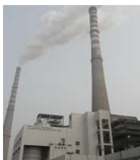
Chongqing Jiulong Power Plant West Plant
