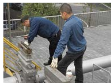
Staff inspecting the equipment at Toutong Station
