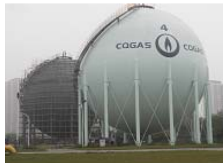
Toutong Natural Gas Station
