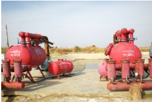
Pumping machine and fertilizer mixing machine (Tacheng)
