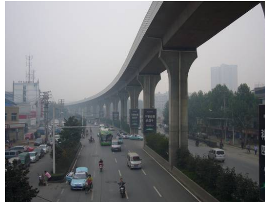
Tracks on viaduct section (Jinghan Avenue)
