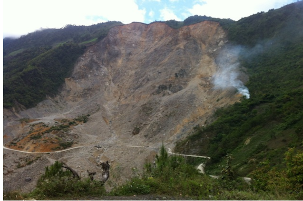
Fig. 2 Current State of the Major Landslide Site at Los Chorros on RN-7W
