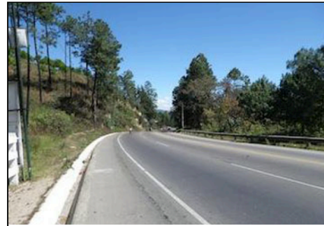
Present State of International Road CA-01W
