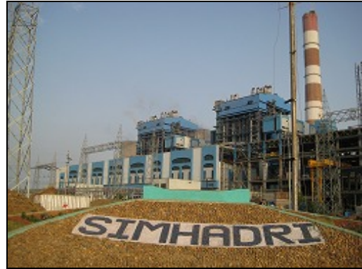
The NTPC Simhadri Thermal Power Plant
