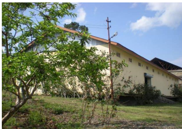
Figure 14: Storage at Bishnupur District
