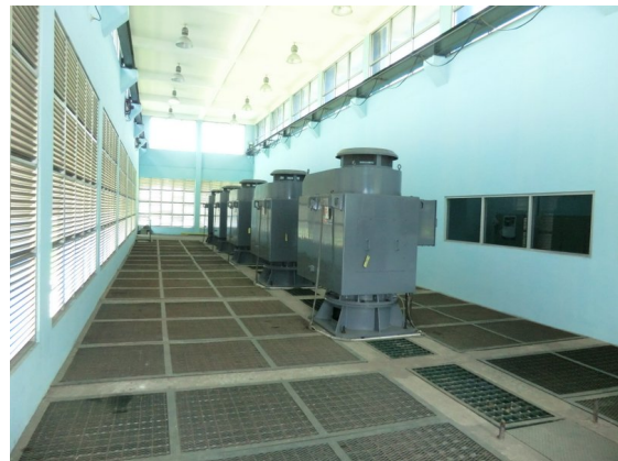
Photo 4 Water Supply: Wonocolo Pump Station
