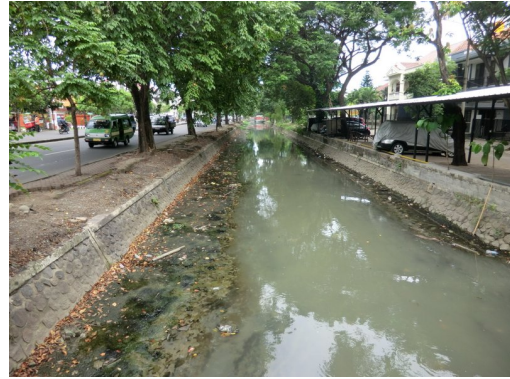
Photo 2 Drainage: Kubong Agung Canal
