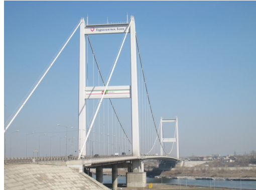
Irtysh River Suspension Bridge
