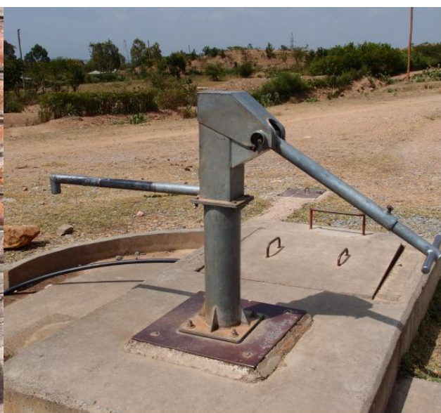
A Manual Standpipe Near the Outlet Channel
