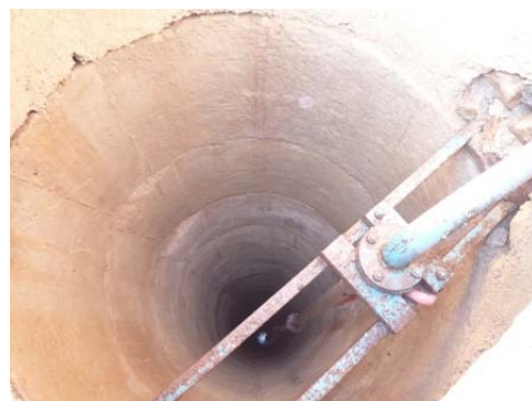
Well excavated in MR-P15
