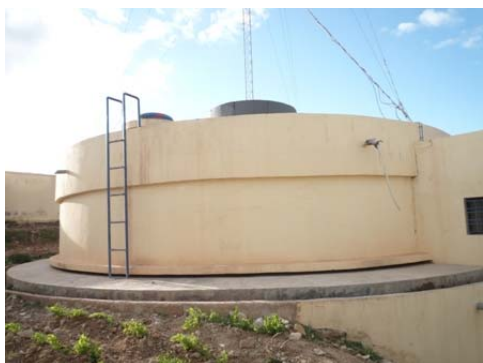
Reservoir constructed in MR-P14
