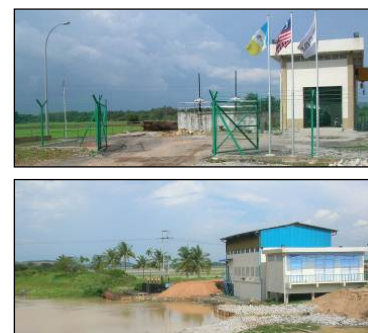
Picture 2: PBA's Water Intake Pump House from the Muda River
