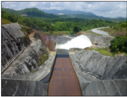
Picture 1: Spillway and Water Release Canal
