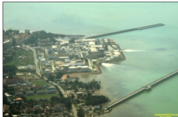
Photo 1: Panorama of TNB Port Dickson Power Station
