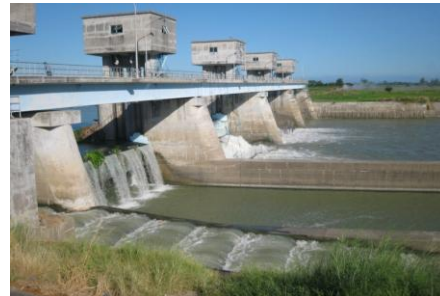
Pampanga Diversion Dam
