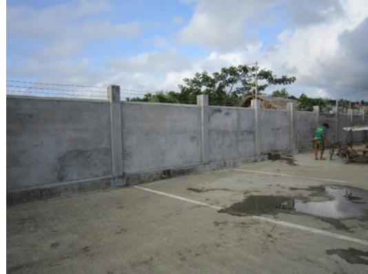
Photo: Repaired part of the ports (Estancia port)
