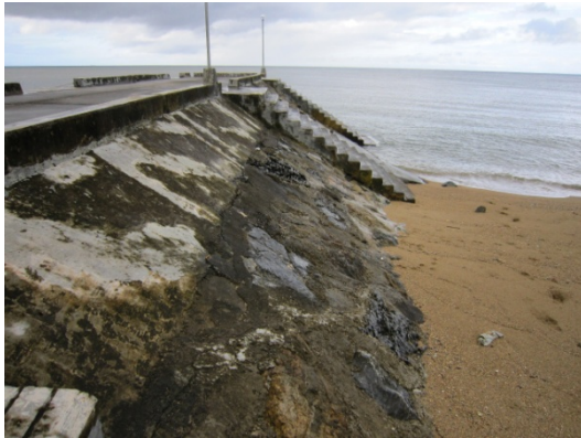
Photo: Repaired part of causeway (Alegria port)
