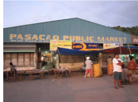
Photo: A market constructed near fishing port (Pasacao)
