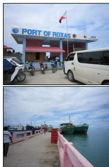
Roxas Port constructed by the Project
