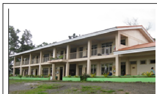
Figure 2. School Building Supported by the Project
