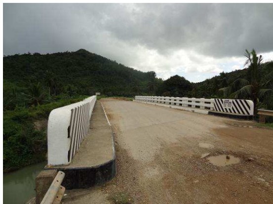
The upgraded bridge (Taytay-El Nido)
