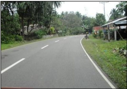
Project Road in Calbiga
