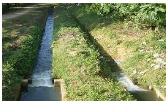
Dual Canal System: The left canal is for paddy and the right canal is for OFC
