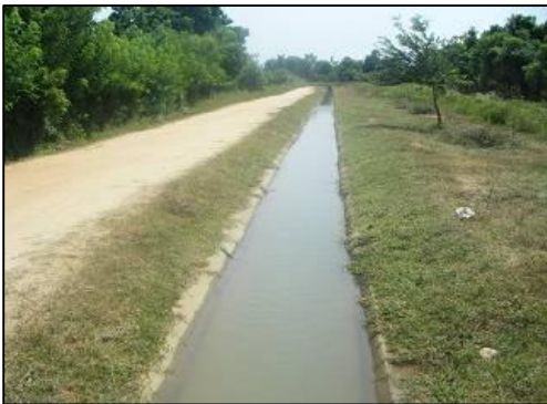
Rehabilitated Irrigation Canal
