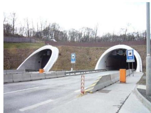
The Tunnel Constructed by the Project
