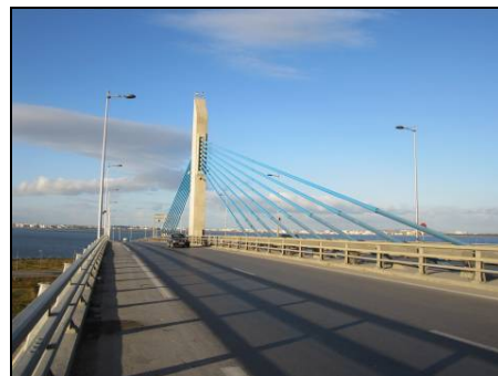
Rades - La Goulette Bridge
