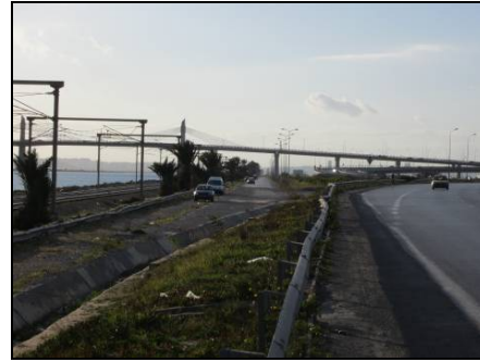
Rades-La Gourette Bridge and Ramps
