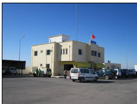
El Jem Maintenance Office
