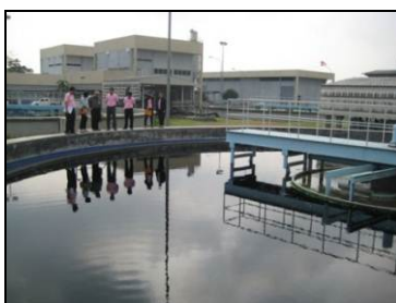
Waste Water Treatment Plant
