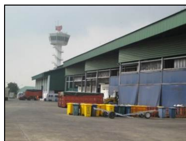
Waste Management Building
