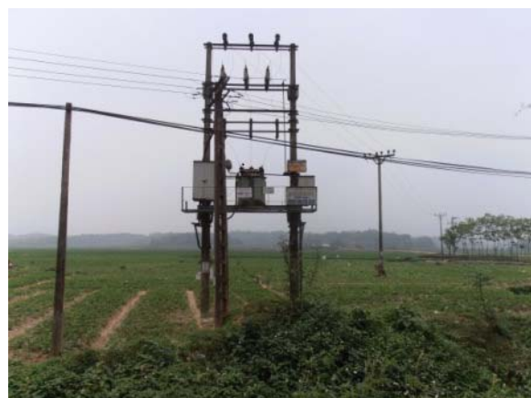
Distribution lines and transformer installed by the project
