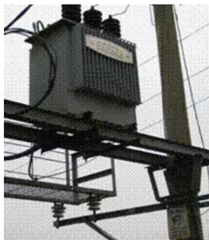
Pole mounted transformer made in Vietnam
