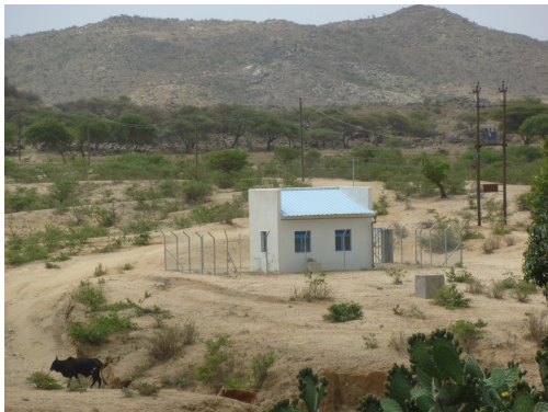
Figure 11: Non-Operational Well and Pumping Facility Due to Electrical System Failure Caused by Lightning (Dekemhare)
