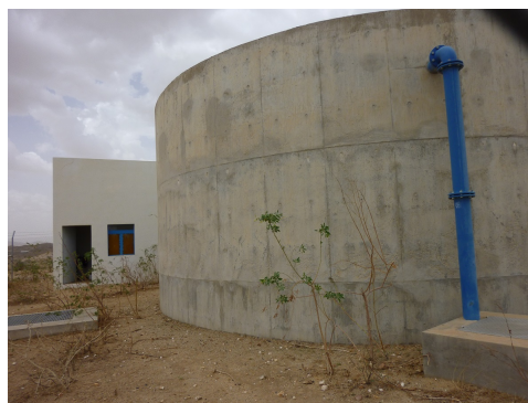
Constructed Reservoir (May-Dima)
