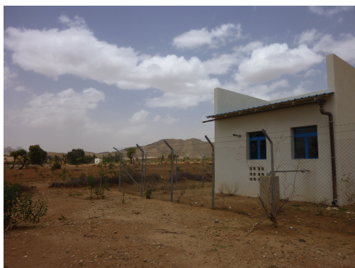
Figure 1: Pumping Facilities (May-Dima)
