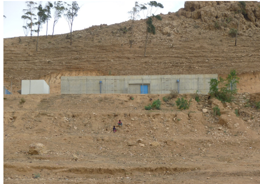
Figure 10: Constructed Reservoir (Dekemhare)
