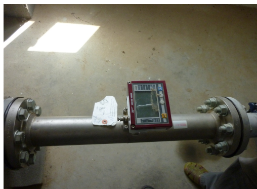
Figure 2: Non-Operating Flowmeter (Dekemhare)
