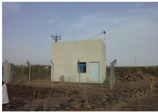
Figure 12: Well and Pumping Facility in Debarwa (it gets flooded in the case of heavy rain as the foundation and the door are built at too low an elevation)
