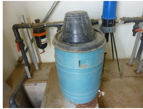
Figure 8: Chlorine Injector
