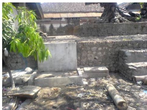
Unrepaired Public Tap
