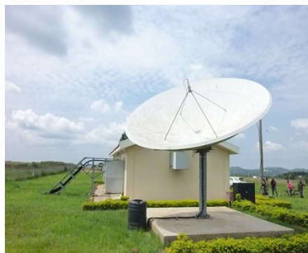
Mawagga MW Radio Transmitting Station
