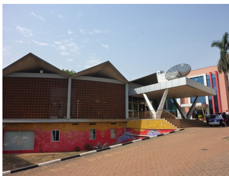
Figure 2: UBC Kampala Broadcast House
