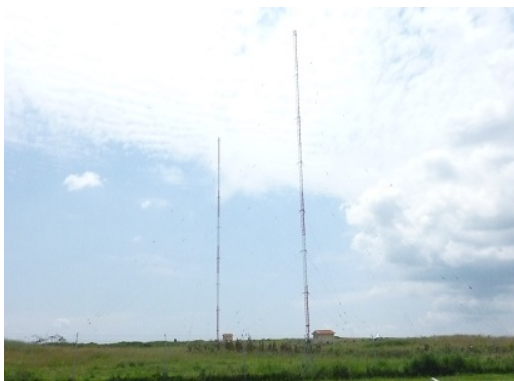
Figure 11: Antenna System at Mawagga Transmitting Station
