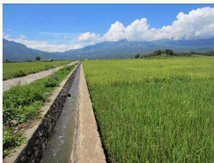
Secondary canal in Ramaskora
