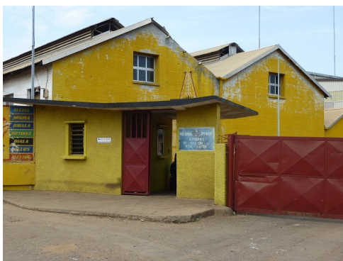
Figure 12: The Exterior of the Kingtom Power Station
