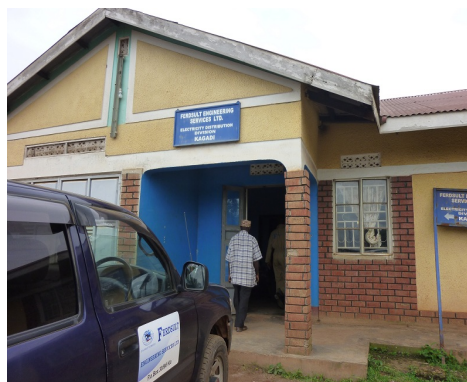
Figure 11: Branch of Ferdsult Engineering Services Ltd. (Kagadi area, Kibale District, Western Region)
