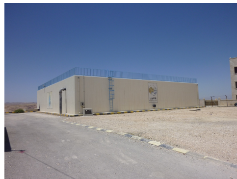
Photo 2: Northern Zarqa Reservoir
