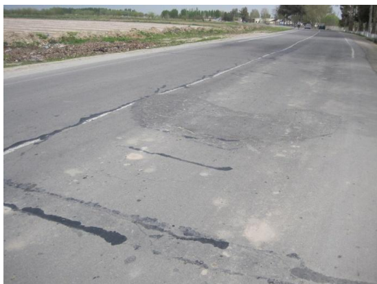
Photo 4: Road surface repaired after damages (Phase I section: surfaces are undulating and the median line is winding.)
