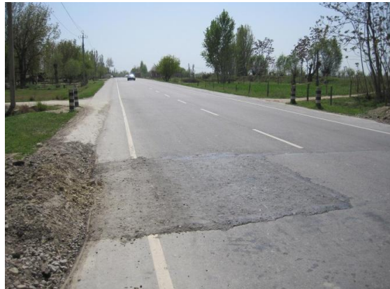
Photo 5: Road surface repaired again after damages (Phase II section: insufficient strength of asphalt)
