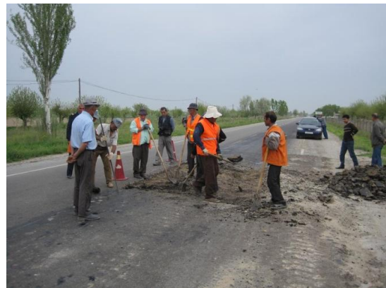
Photo 3: Subsequent repair work on a spot once repaired by SEHM (Phase II section)
