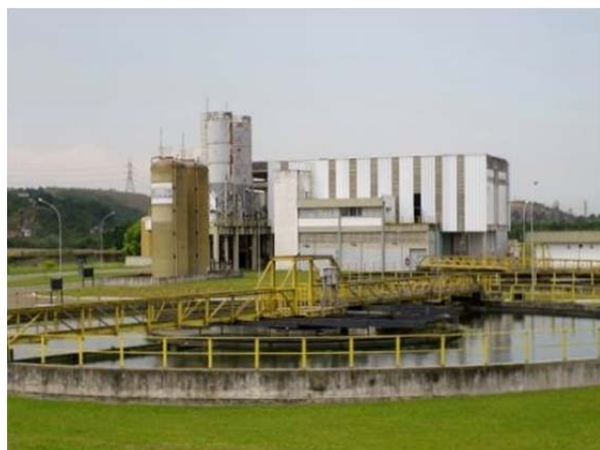
Primary Treatment Facility (Sarapui WWTP)
