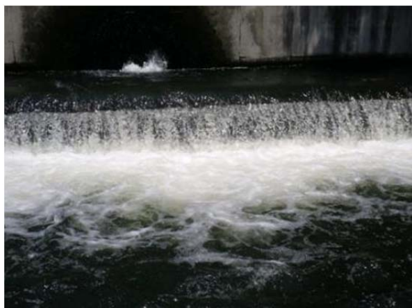
Treated Water Before Discharge (Alegria WWTP)
