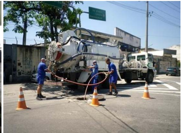
Maintenance works of sewer
