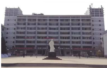
Teaching Building constructed using funds from the Chinese side (GCTCM)
