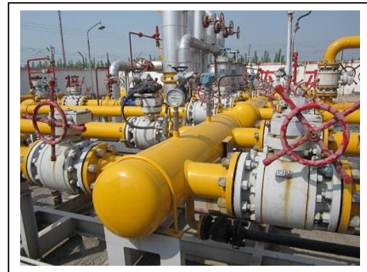
Figure 17: Piping in a gate station (Jiaozuo)
