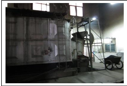
Figure 4: Coal boiler facility (Xinyang)
