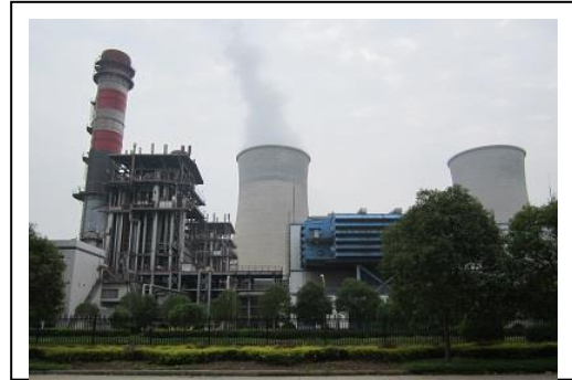
Figure 5: Thermal power plant (Xinyang)
