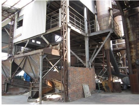
Figure 17: Coal-fired boiler before conversion (Ma'anshan City)
