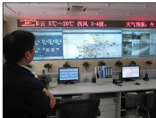
SCADA System (Hefei City)
