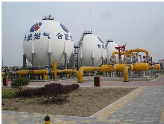
Figure 19: Spherical natural gas holders (Hefei City)
