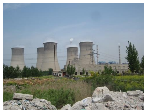
Figure 6: Thermal power station (in Huainan City)
