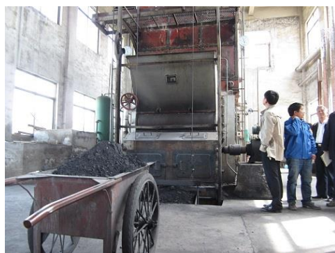
Figure 5: Coal boiler facilities (in Chuzhou City)
