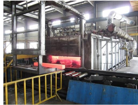
Figure 18: Natural gas furnace after conversion (Ma'anshan City)
