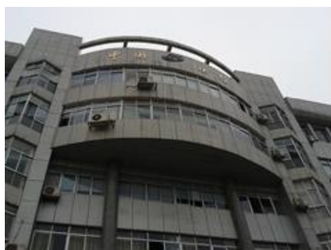
Figure 1: Exterior view of the Xiangtan City CDC
