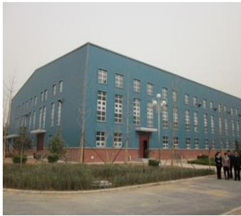
Figure 6. A building housing a water purification plant (Tongchuan)
