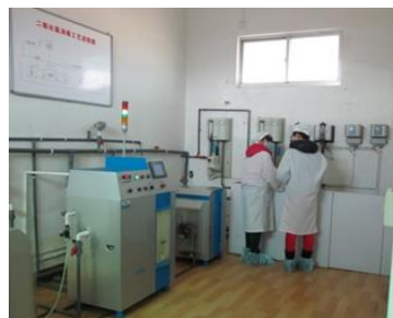
Figure 4: Chlorine Dioxide 38 Generation Facility (Fuping County)
