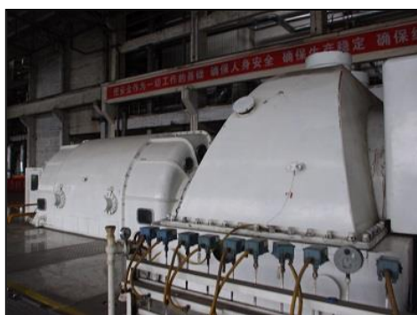
Heat supply/electricity-generating turbine installed
