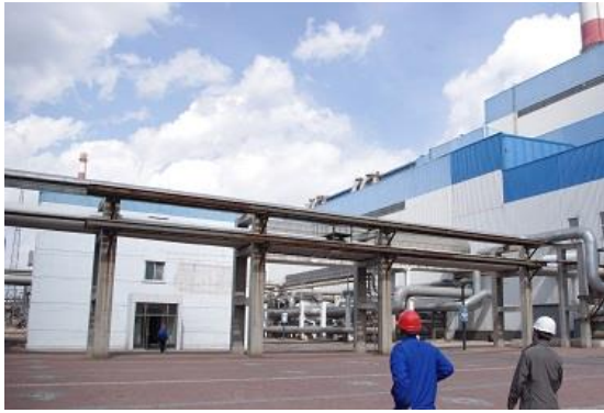
Figure 5: The Air around the Shenyang Thermal Power Plant
