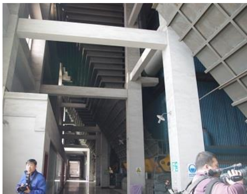
Figure 1: Taiyuan Jie Central Heat Supply Boiler
