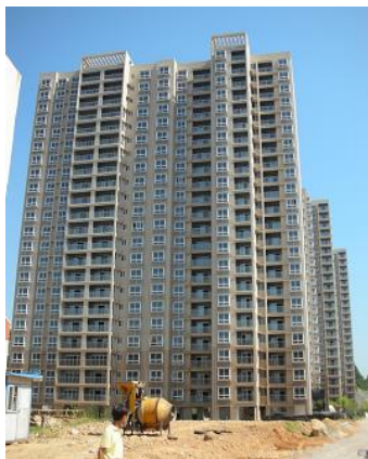
Figure 3: “Resettlement Residence” in Changsha City
