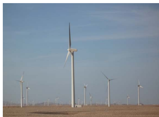
Wind Power Plant Constructed by the Project
