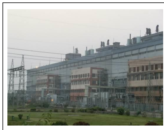
Bakreswar Thermal Power Station
