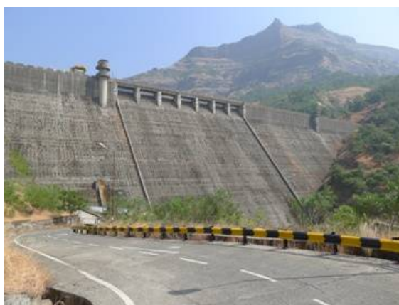
Ghatghar Pumped Storage Hydropower Station
