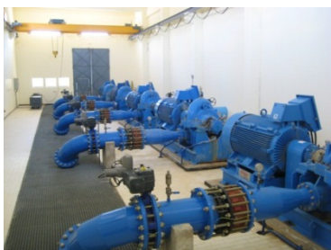
Pumping Station No. 2
