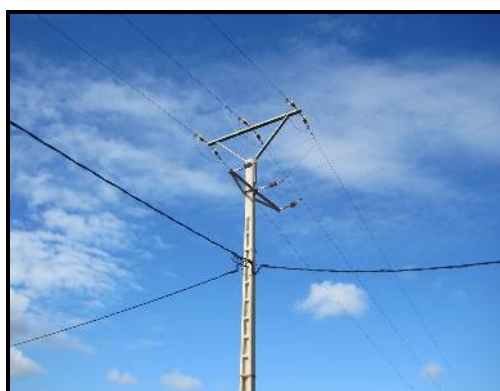
Distribution lines constructed under the project (Essaouira Province)
