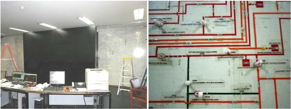
Distribution Control Room (left; large display units not in use, right; manual display unit)
