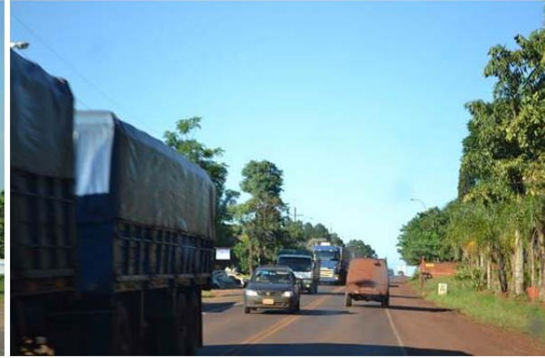
Track for Grains (Road Section 4)
