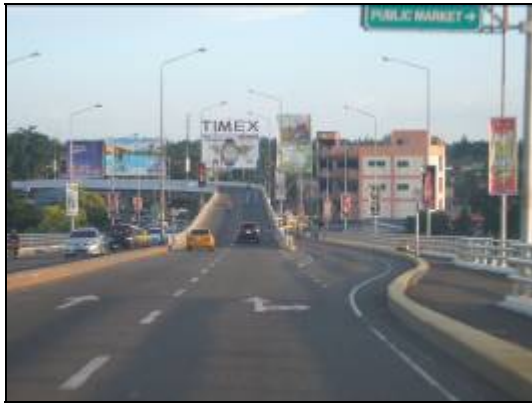
Left-turn Ramp at Mactan side Second Mactan Bridge
