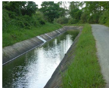
Constructed Main Canal
