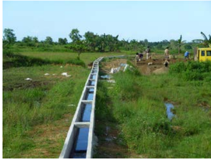
Figure 12: Concrete-Lining of Tertiary Canal
